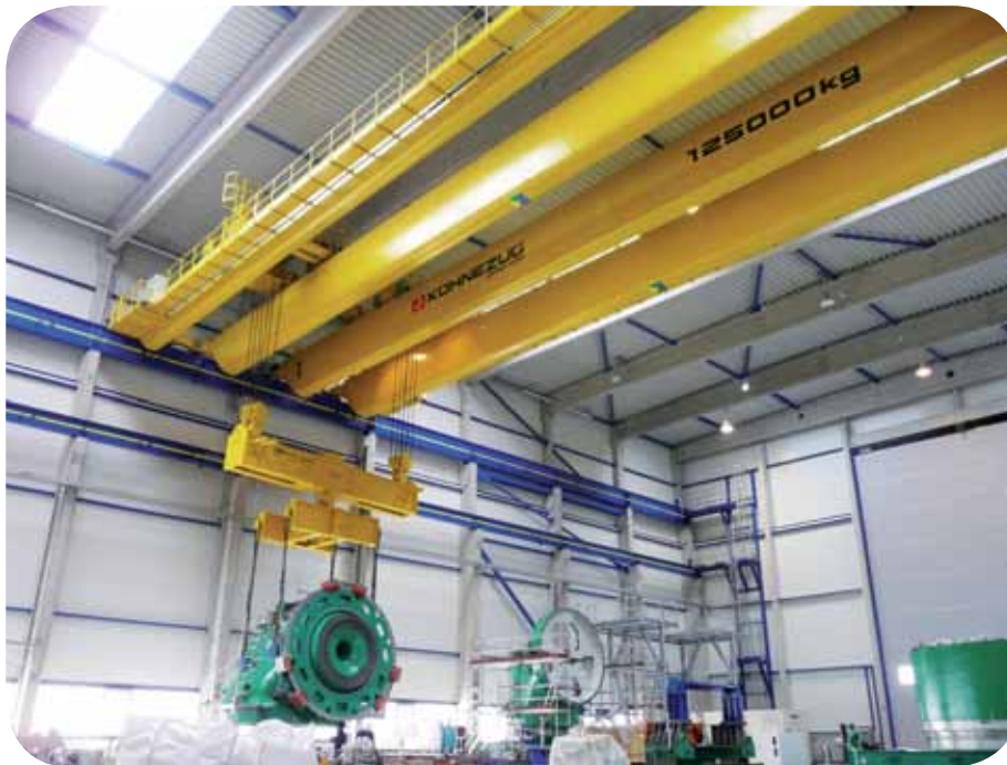
2 x 125 t / full tandem / offshore wind turbine
