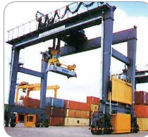
RTG Container Handling Crane
