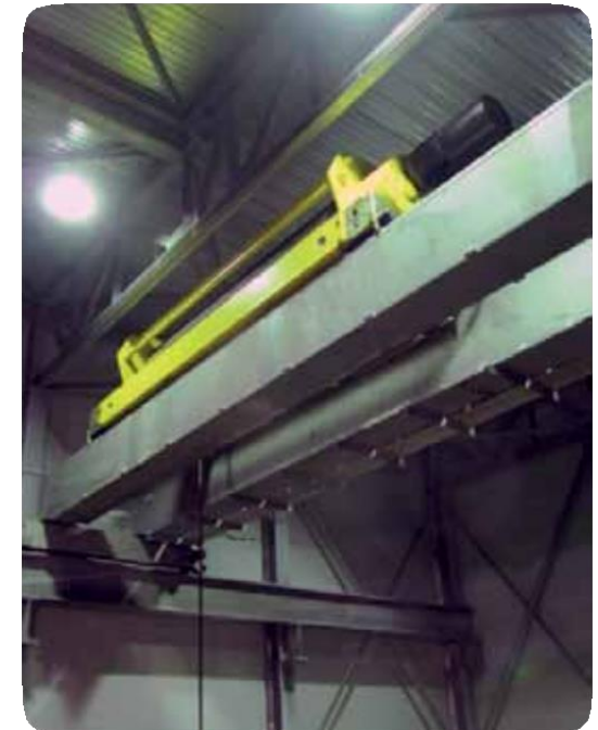
25 t / 190 m HOL / 100% true lift by self adjusting automated trolley
